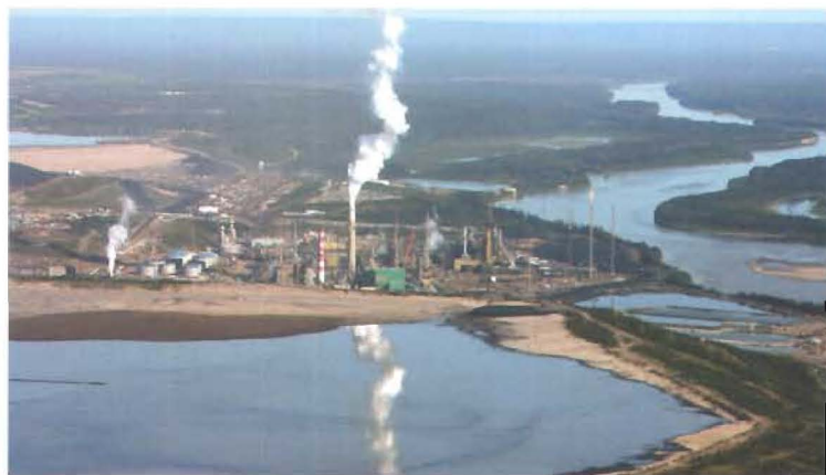
Figure 11.8 The mining and petroleum industries use large volumes of water. In Alberta's Athabasca River basin, hot water is used to separate the oil from the oil sands deposits.
