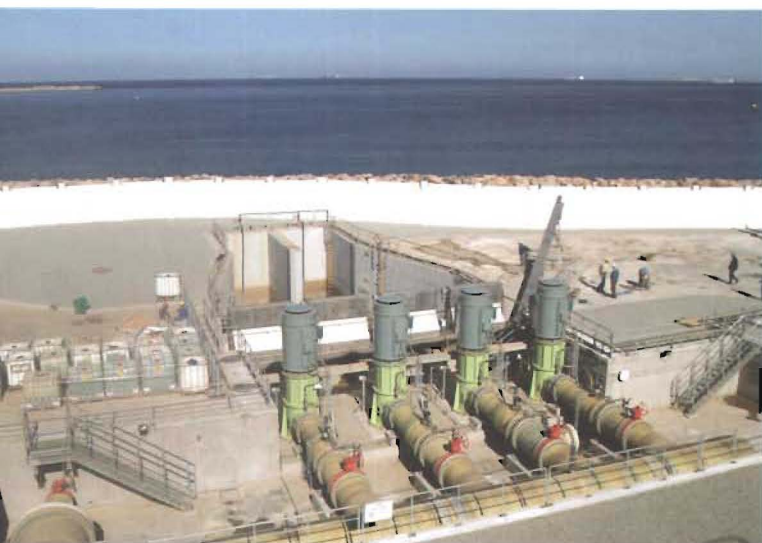
Figure 12.18 Africa’s largest desalination plant is in Algeria. It can produce 200 000 m 3 of drinking water daily from the Mediterranean Sea.
